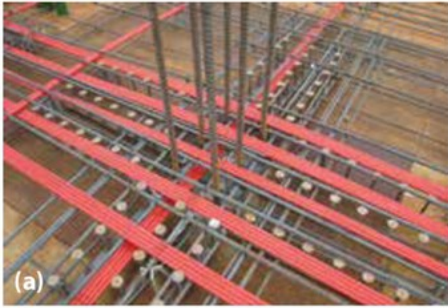
Figure 2. Two-way slab construction with unbonded and bonded post-tensioning tendons. (a) Slab construction with unbonded tendons. Neither ACI nor EC2 requires a strength check at the initiation of cracking (P998). (b) Slab construction with bonded tendons ACI requires a strength check at the initiation of cracking. EC2 does not (P999).
