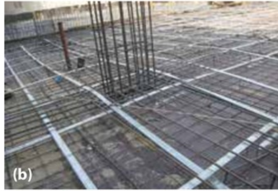
Figure 2. Two-way slab construction with unbonded and bonded post-tensioning tendons. (a) Slab construction with unbonded tendons. Neither ACI nor EC2 requires a strength check at the initiation of cracking (P998). (b) Slab construction with bonded tendons ACI requires a strength check at the initiation of cracking. EC2 does not (P999).
