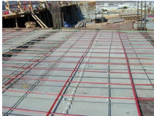
FIGURE 4.8.4-4 Disadvantageous Slab Tendons between Post-Tensioned Beams (P326)
