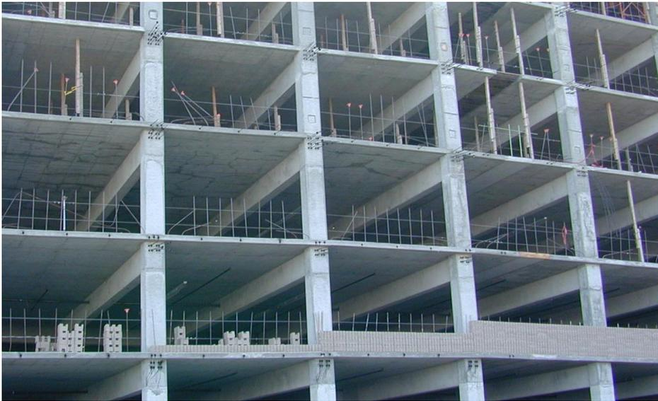
FIGURE 1 Post-tensioned beam and slab construction with temperature tendons in the slab between beams. The stressing pockets of three temperature tendons at the edge of the slab are visible.(P355)
