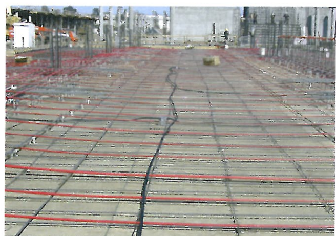
(b) Distributed tendons placed parallel (P424)
