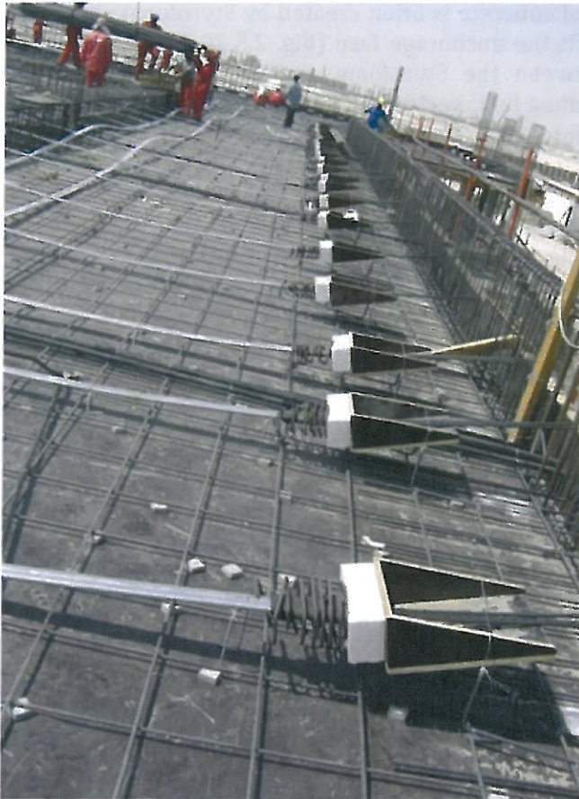
FIGURE 2.5.2C-3 Row of Stressing Pans Next to Wall (P181)
