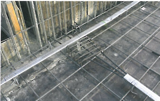
FIGURE 2.5.2C-4 Anti-Bursting Reinforcement behind Anchorage Device (P183)
