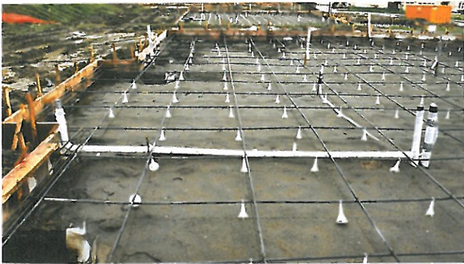
Fig. C.1-2—Ground-supported slab using unbonded tendons.
