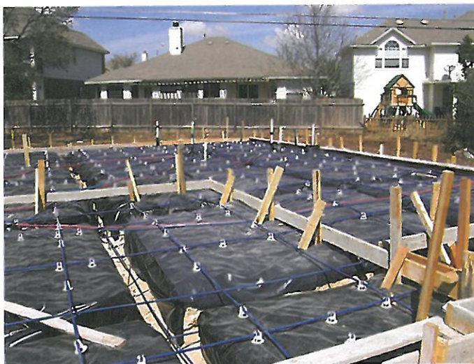
(b) Ribbed slab ready to receive concrete.
