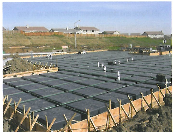
Fig. C.10-3—Ground-supported waffle slab construction. (courtesy CONCO)
