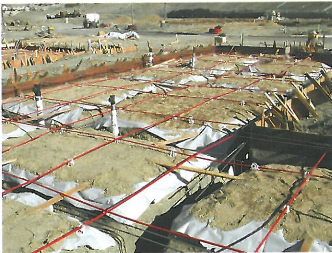
(a) Slab with drain sand over moisture barrier.
