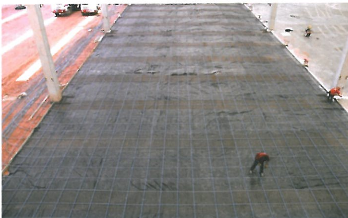
Fig.—C.1-4 Industrial ground-supported slab.
