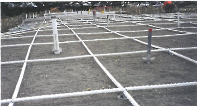
Fig. C.1-3—Ground-supported slab using bonded tendons.
