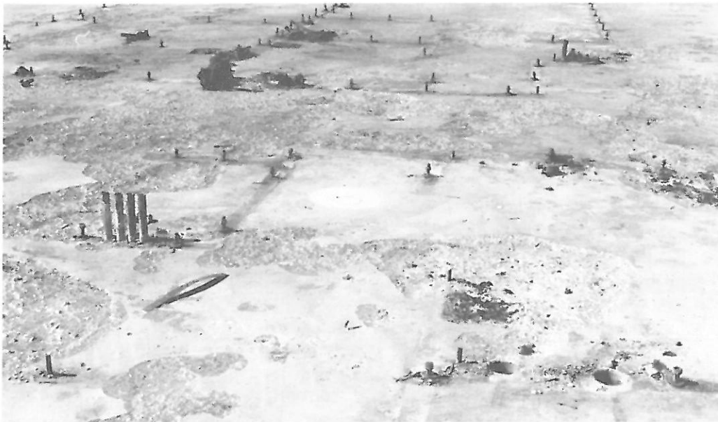
PICTURE 1: CONCRETE SPALLING IS MORE PRO- NOUNCED AT MIDSPANS AWAY FROM COLUMNS AND WALL SUPPORTS.
