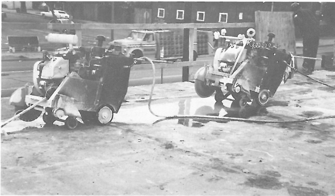
PICTURE 9: EQUIPMENT USED TO SAW CUT SLAB.
