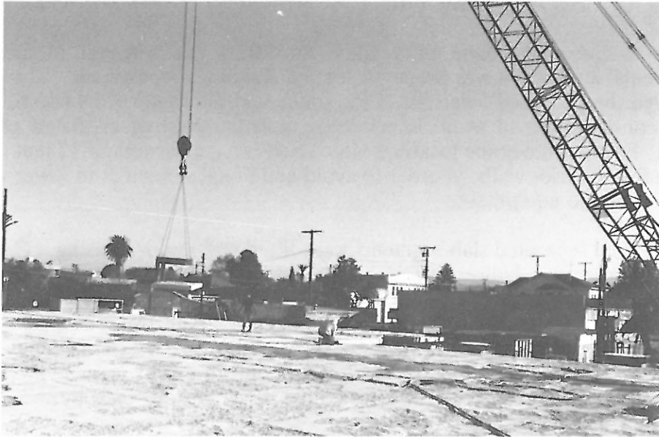
PICTURE 21: THE LIFTED SEGMENT IS BEING REMOVED.
