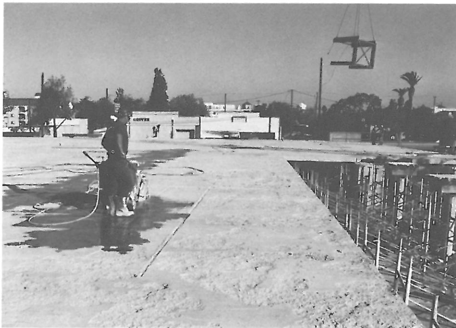
PICTURE 20: THE C-HOOK IS BEING LOWERED TO PICK UP A SEGMENT WHICH IS CUT AWAY.
