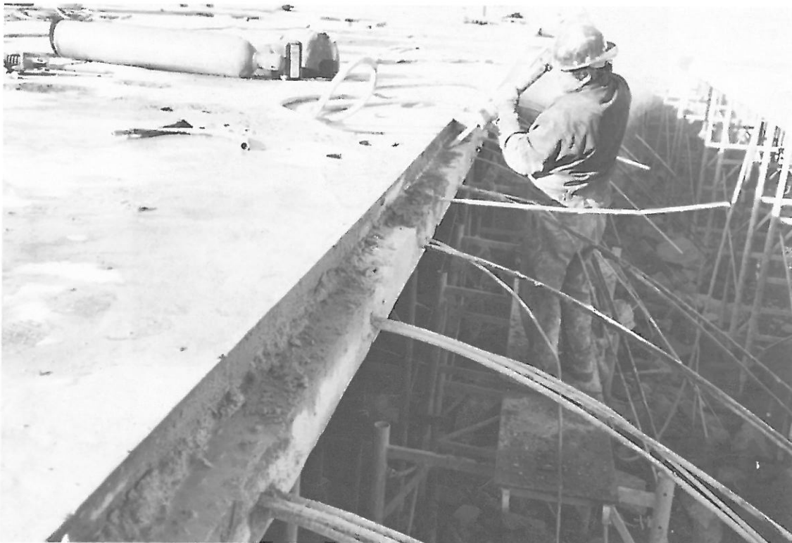
PICTURE 26: A SUPPORT LEDGER IS CUT OUT OF THE SLAB EDGE.
