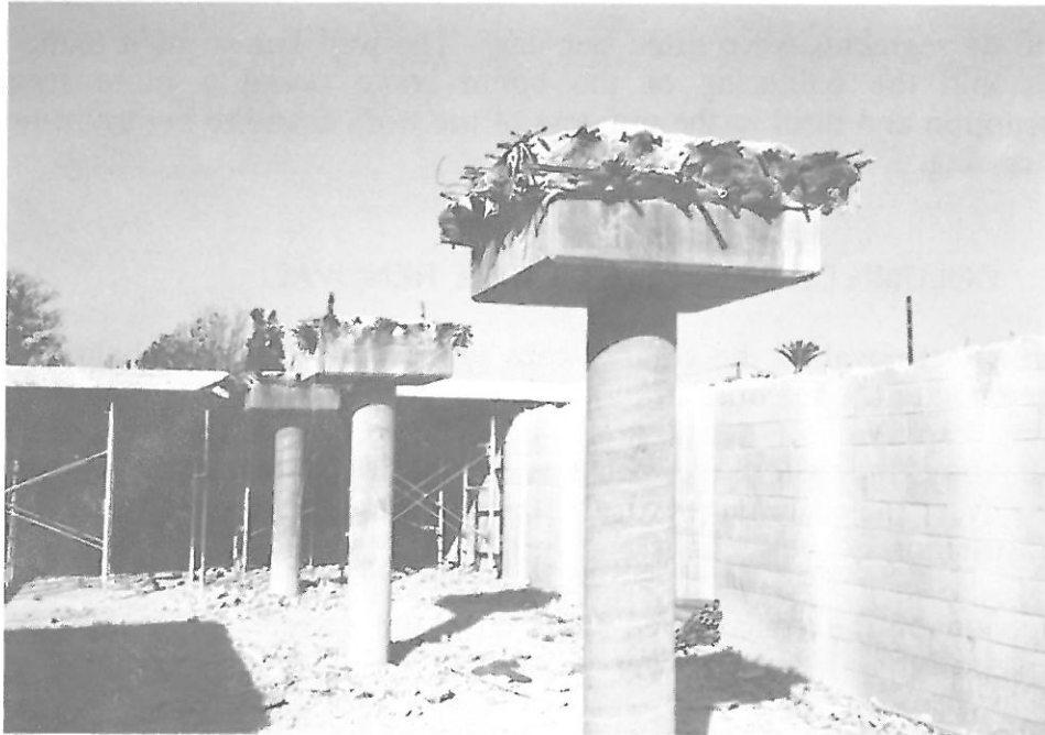
PICTURE 23: EXPOSED COLUMN CAPITAL AFTER REMOVAL OF SLAB.
