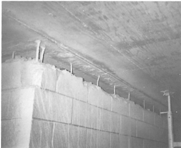
PICTURE 19: THE WALL CONNECTION TO THE SLAB WAS CHIPPED OUT.
