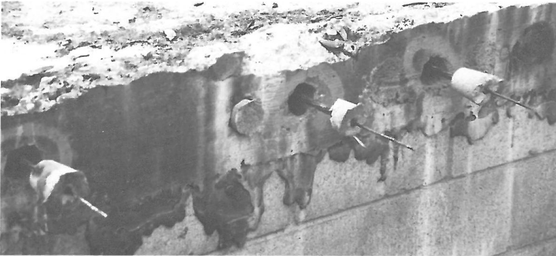
PICTURE 14: OBSERVE THE KERN WIRE EXTENSION BEYOND THE INTACT GROUT PLUG.
