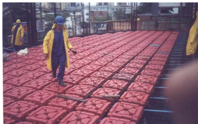
(b) Construction view
