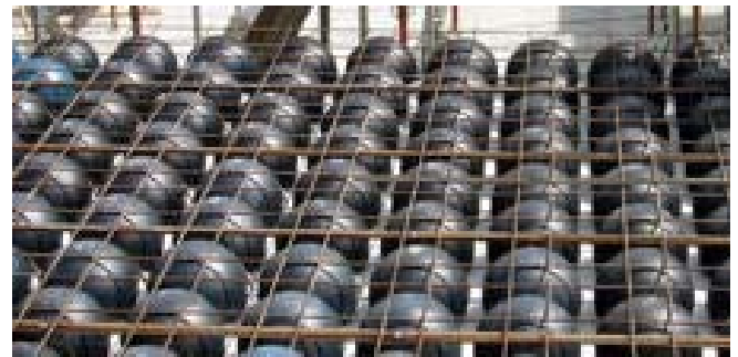
(b) View of a voided slab in construction
